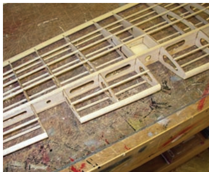
After the main wing structure is completed, remove the sections shown here for the engine nacelle structures.
